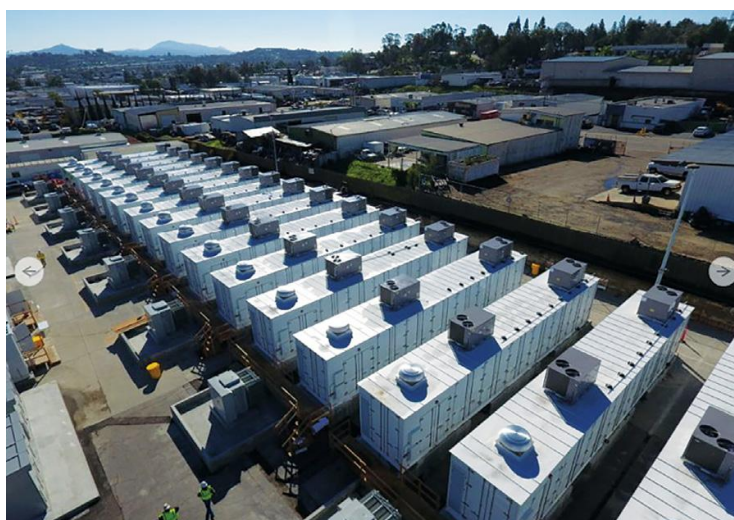
Figure 8. In 2016, AES Energy Storage deployed the largest of these farms for San Diego Gas & Electric, connecting 400,000 individual batteries into 24 containers to store 120 MWh of electricity for up to four hours. From Power Engineering, 2019. Implications of lithium-ion storage transformation [ https://www.power-eng.com/2017/11/15/implications-of-a-lithium-ion-storage-transformation/#gref ].
